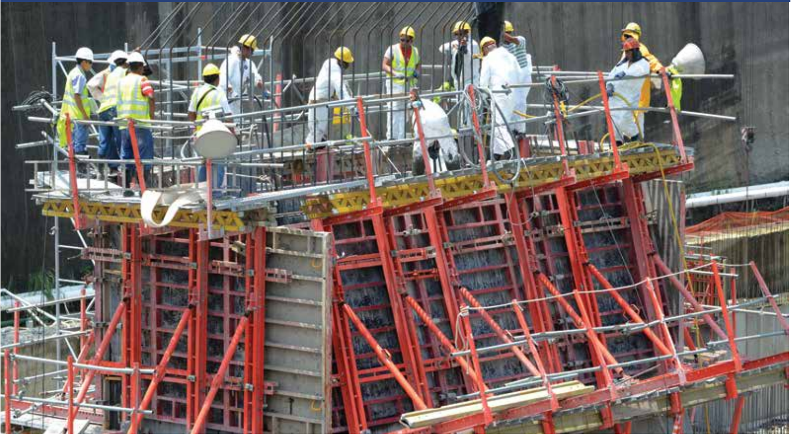
Atlantic locks builders.
